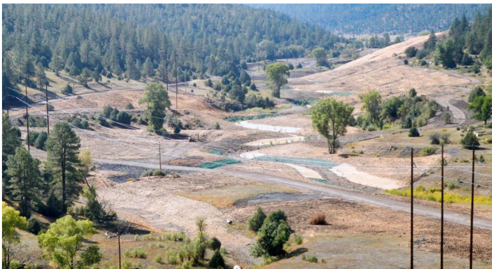
Figure 22. Completed geomorphic reclamation and stream restoration at Swastika.
