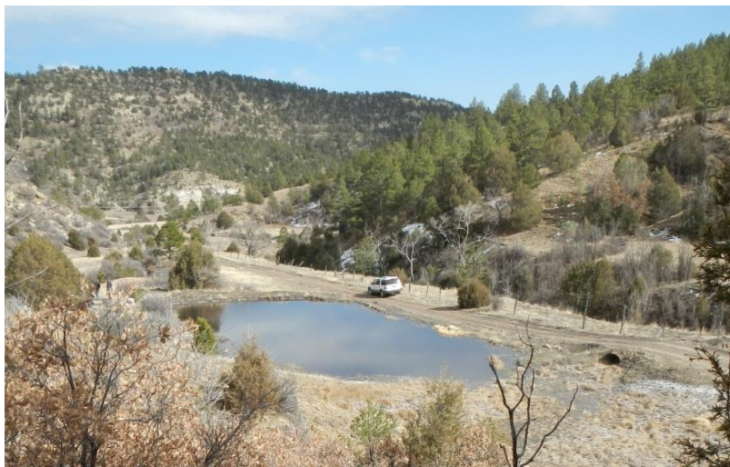
Figure 2. Wildlife pond and outlet culvert at Dutchman Canyon.
