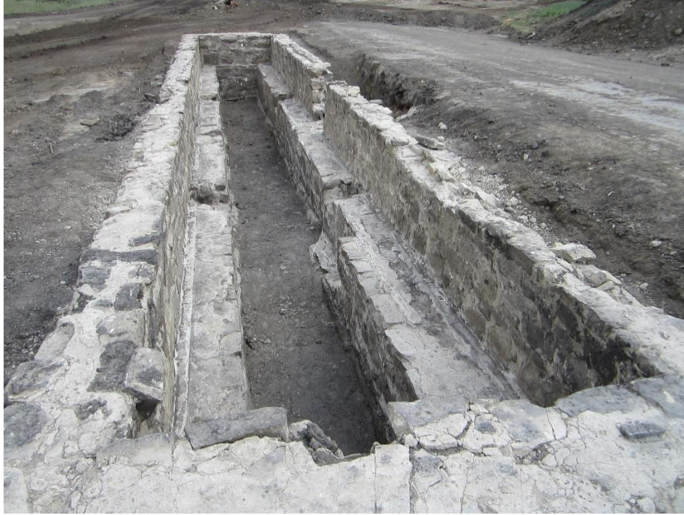
Figure 14. Buried railroad service pit encountered during channel excavation.
