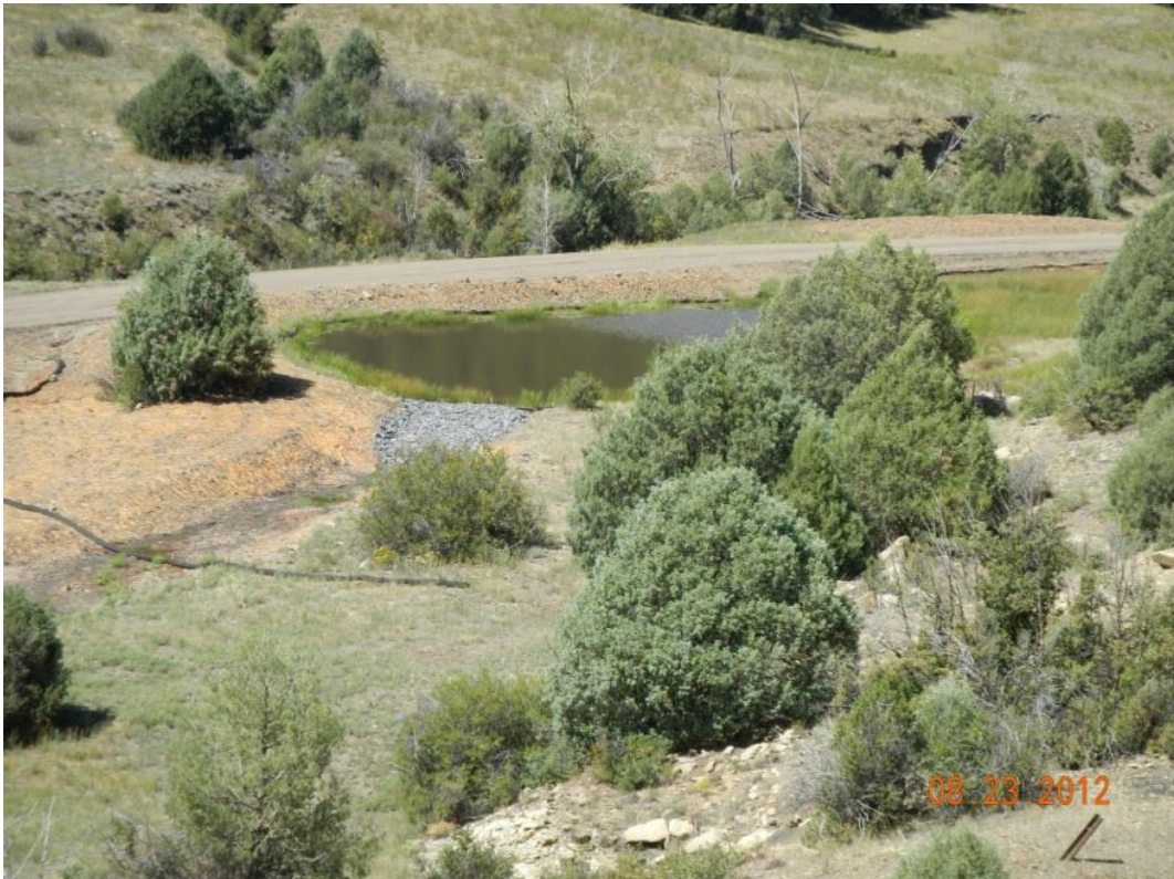
Figure 24. Embankment improvement increases freeboard, provides a spillway, and directs outflow to a new salt-tolerant wetland.
