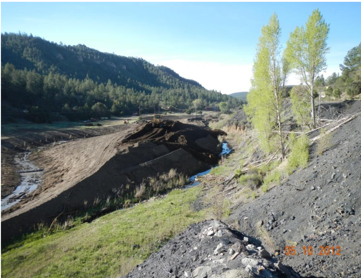
Figure 17. Realigned and restored channel construction.
