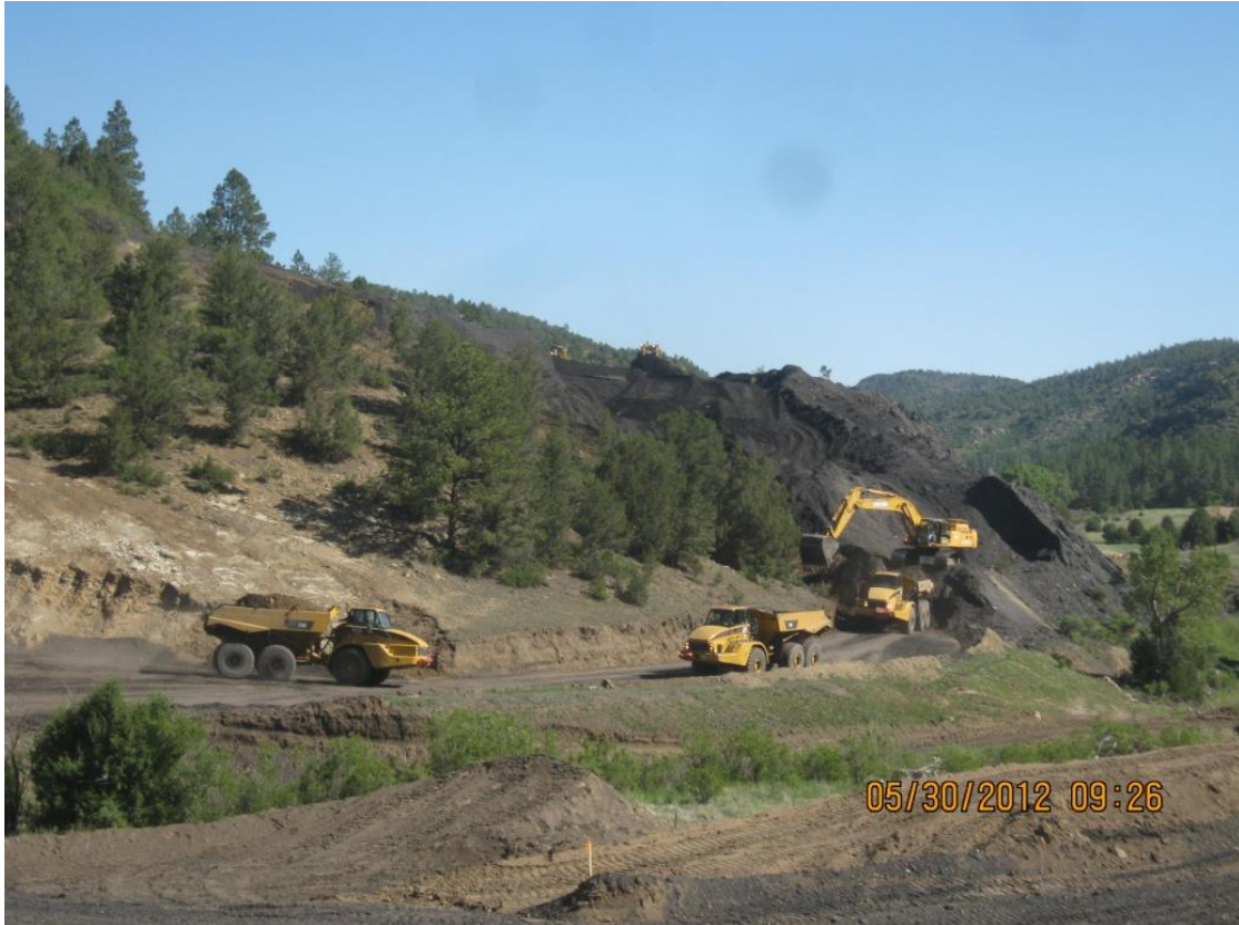
Figure 16. Removing coal waste to combination soil borrow/repository areas.
