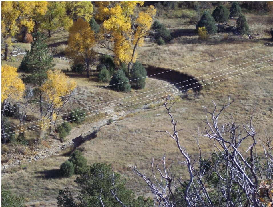
Figure 10. Undisturbed reach in Coal Canyon showing variable side slopes for channel banks.
