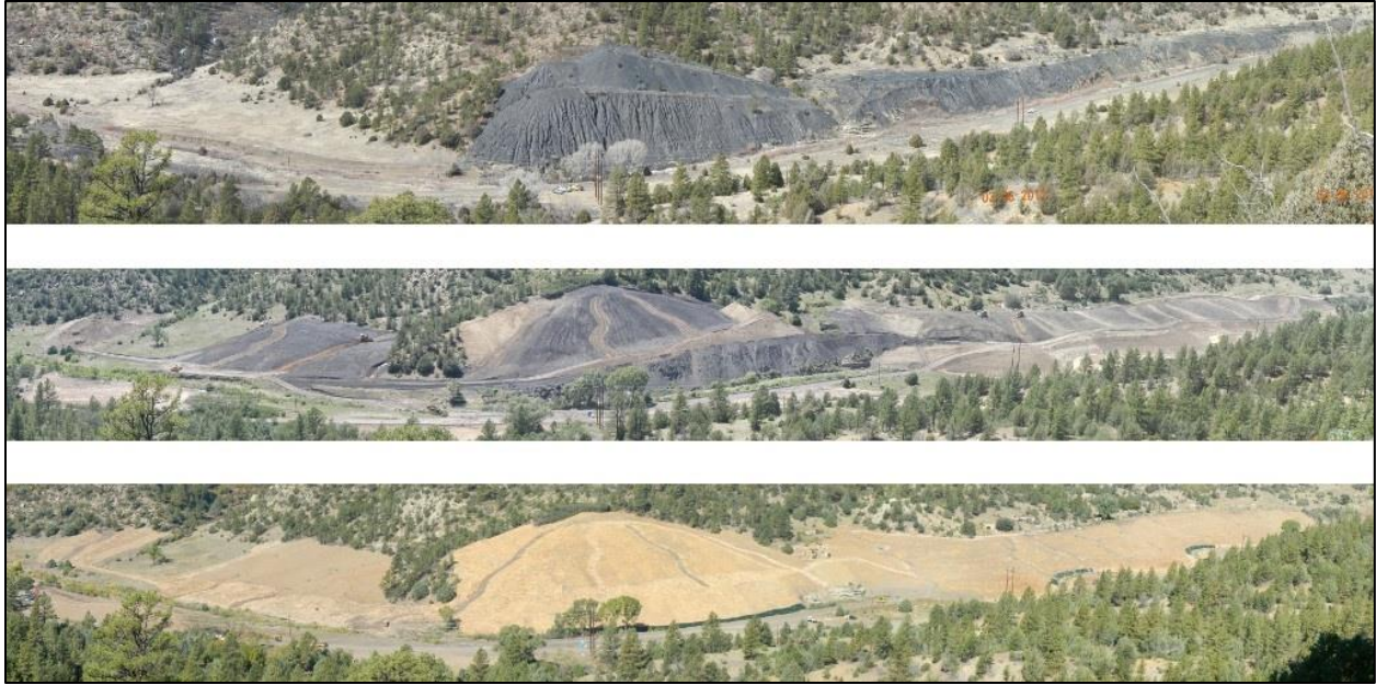
Figure 20. Coal waste reclaimed in geomorphic landforms at Swastika.
