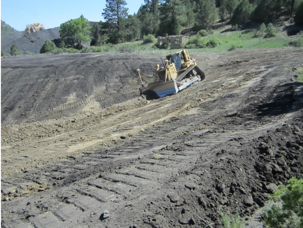
Figure 15. Landforming with GPS machine control.
